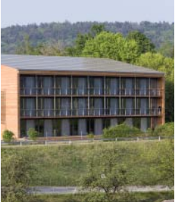
Figur 13: Marché International Support Office, Kempptthal
