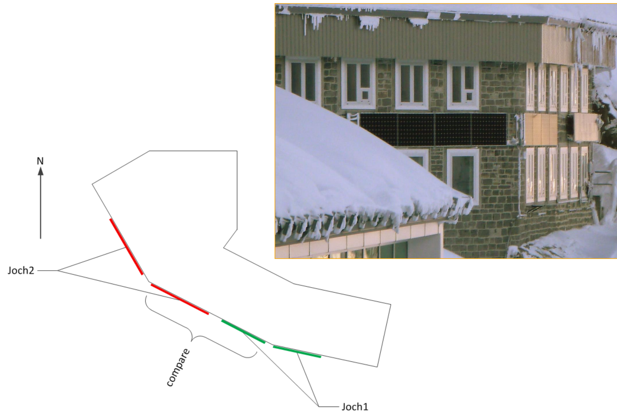
Fig. 2: Position of the PV modules on the Jungfrauoch research building (Joch 1 (right): PV-installation 1993; Joch 2 (left): PV-installation 2014).
